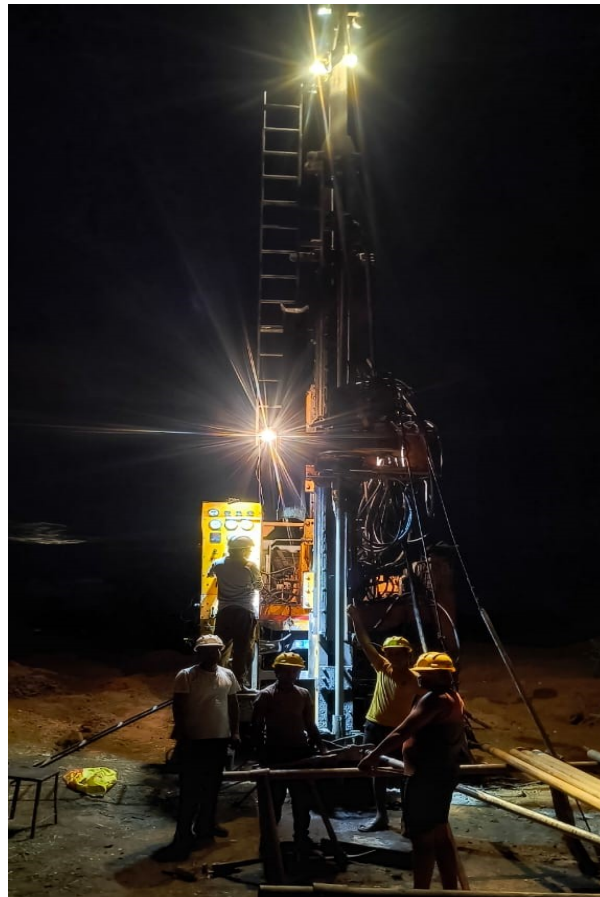
Photo-13.2 Photograph of KDR-1000 drill Rig under operation in night shift at MPN-05
